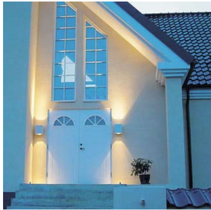
Fasadbelysning, Helsingborg Superlight Twin
